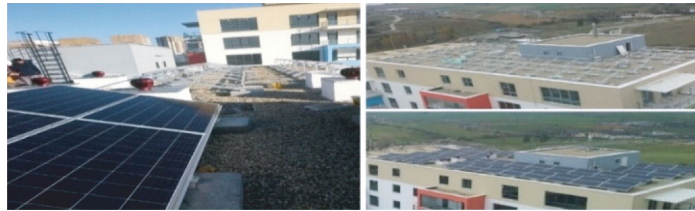
FIGURE 4: Project installation stages.
